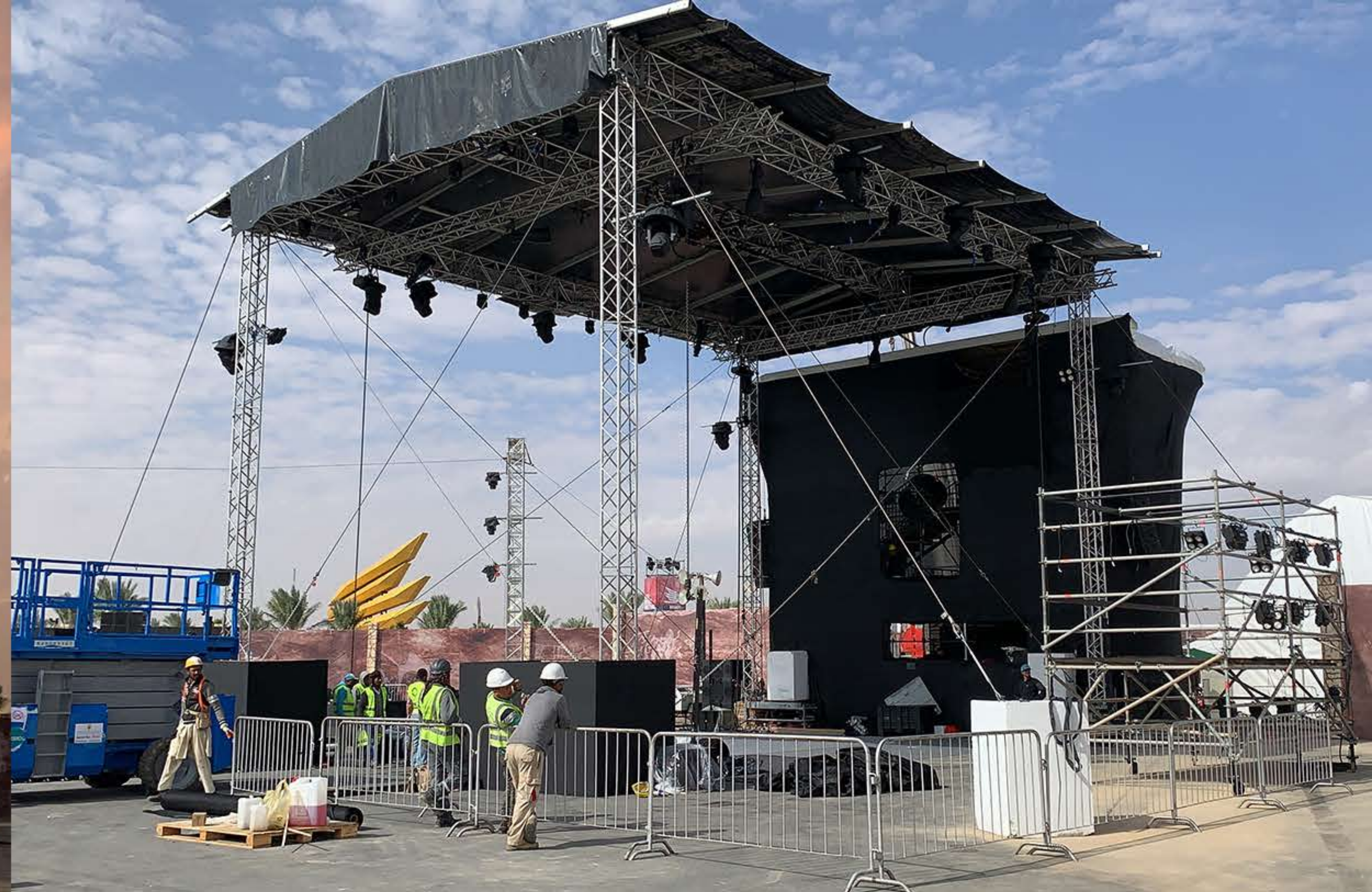
Fuerta Bruta stage 13m x 12m x 10m (h) ground support stage, with suspended water pool, supporting a live dynamic load of 1 tonne.
