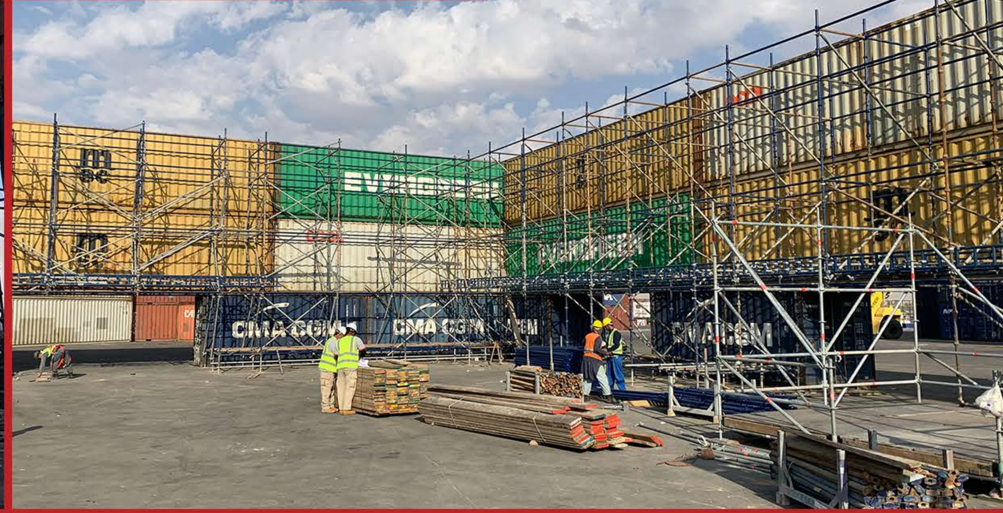
Stage 3 & Stage 4 Individual music zones, with scaffold enclosures for supporting LEDs. DJ Bandroofs installed by AES.
