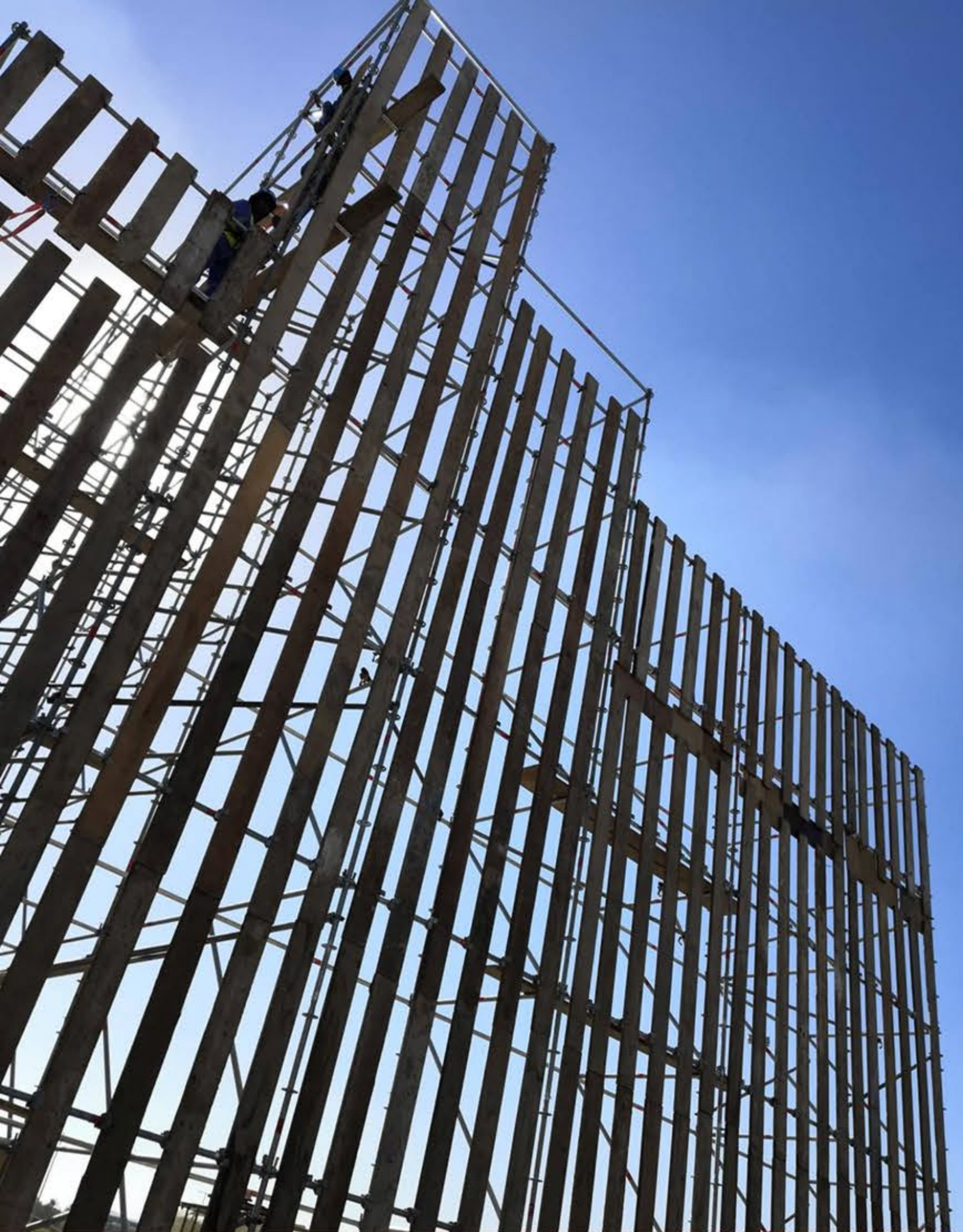
Scaffold boards attached to steel
