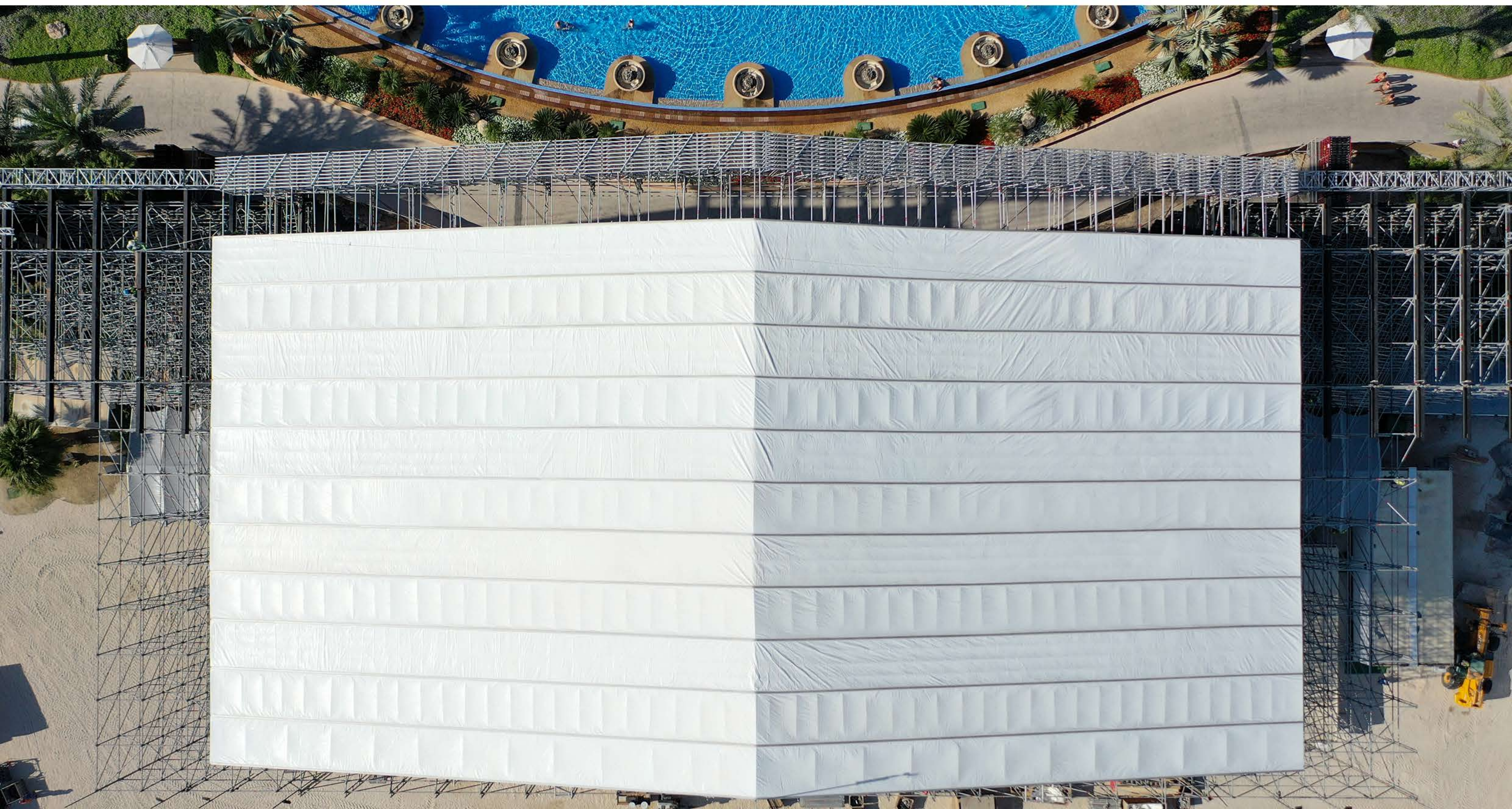
FLAME RETARDANT ROOF SKINS INSTALL OFFERING A WEATHER PROOF STAGE COVER
